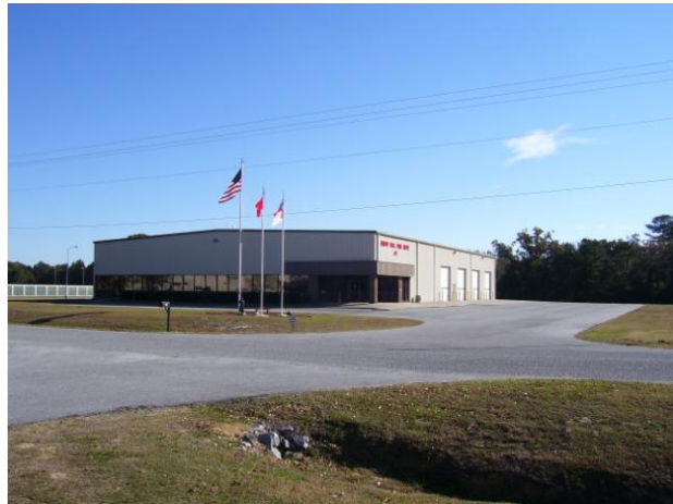
Snow Hill's fire department is located on Carolina Drive with easy access to Kingold Boulevard
