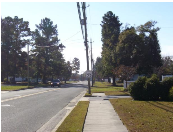
Abrupt end to sidewalk on SE 2 nd St.
