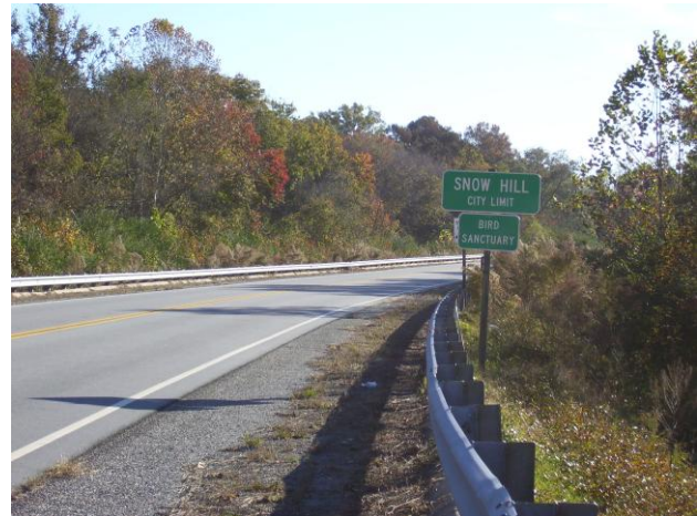
The greenway trail network would follow alongside NW Second Street (shown) into the Central Business District.
