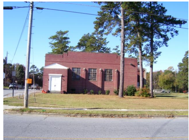
The town would like to acquire and renovate this building for a multi-purpose community center.
