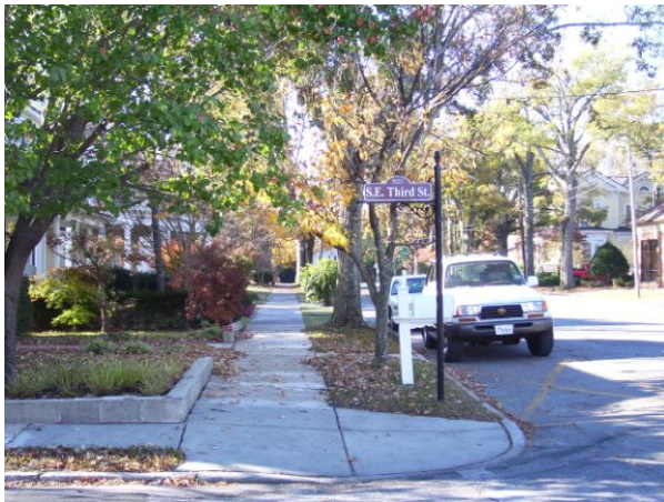
Existing Sidewalk Conditions (Greene St and SE 3 rd Street in CBD)
